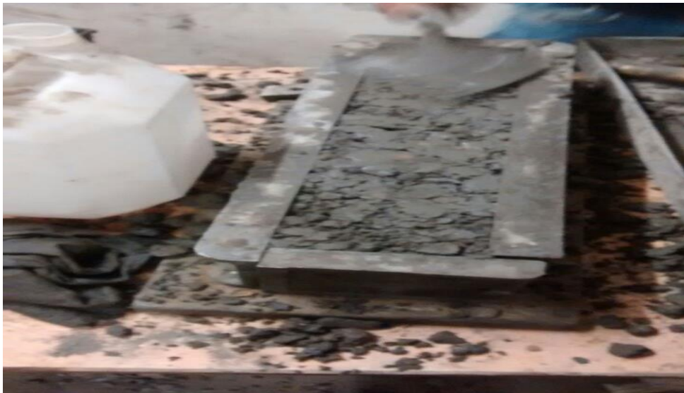
Figure 3.12: Casting of beams
