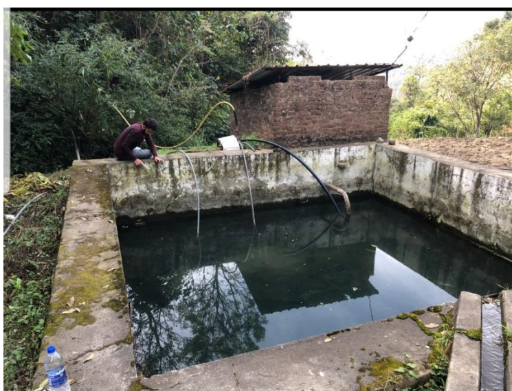
Fig. 4.17: Storage Tank of Wakna
