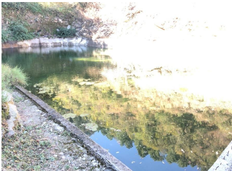
Fig. 4.13: Open Storage Tank of Bisha
