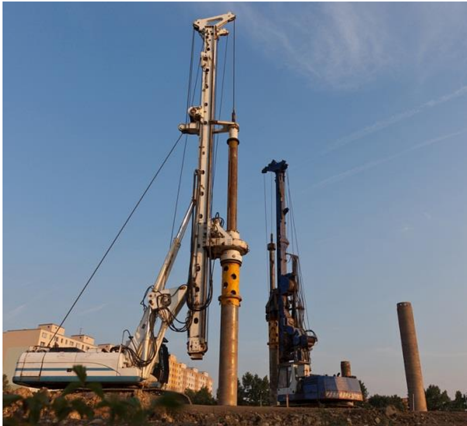
Fig. 6.6.4: Pile driver
