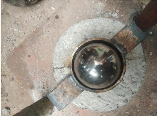
Crack initiation at 1%
