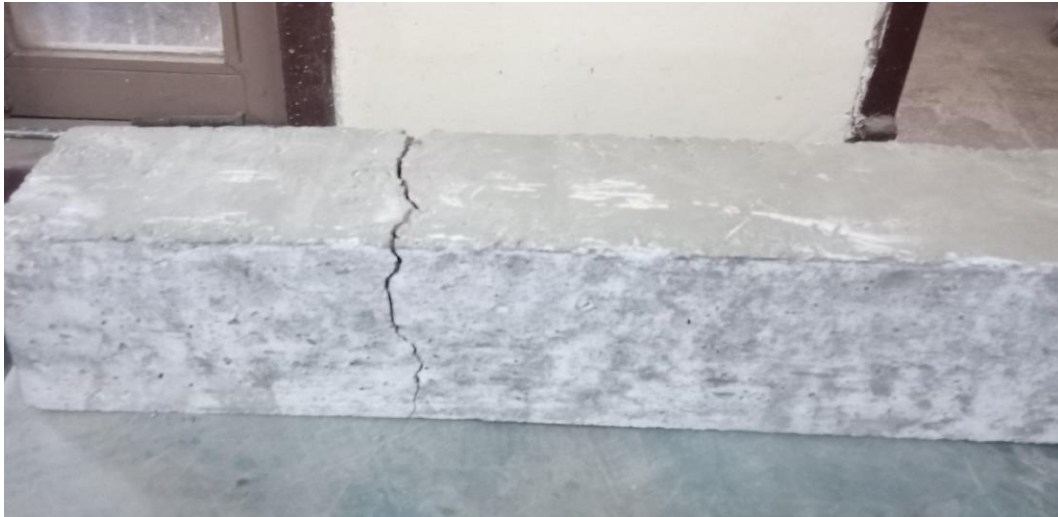
Figure 4.6 Failed beam under flexural loading
