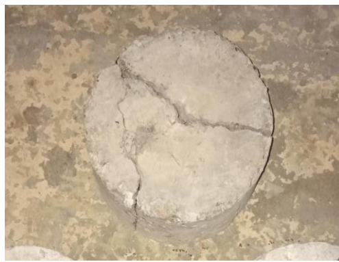
Crack failure at 1.5%
