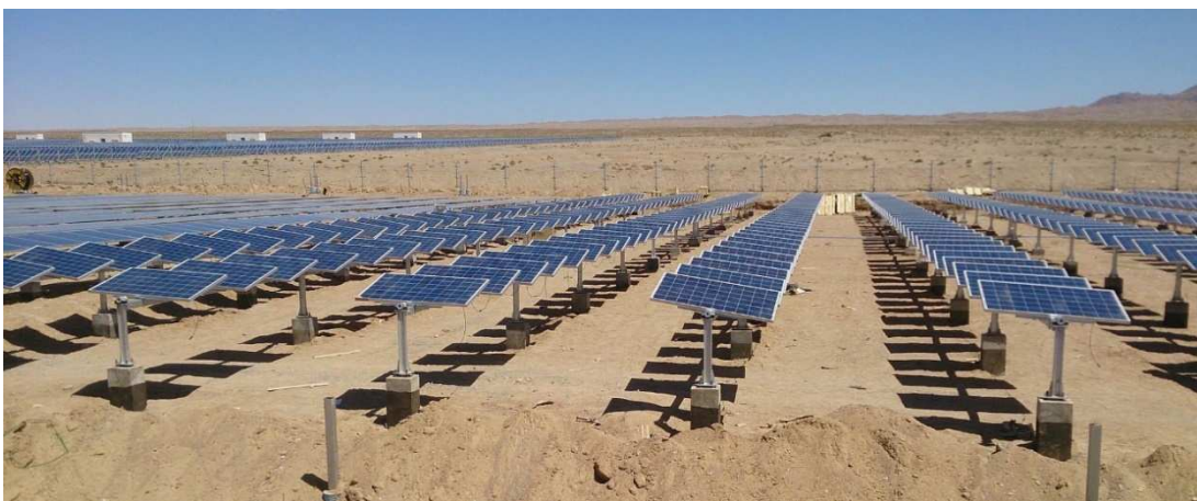
Figure 3.1: Horizontal Single Axis tracker with Tilted Modules in Xitianshan, China. Commissioned in July 2014
