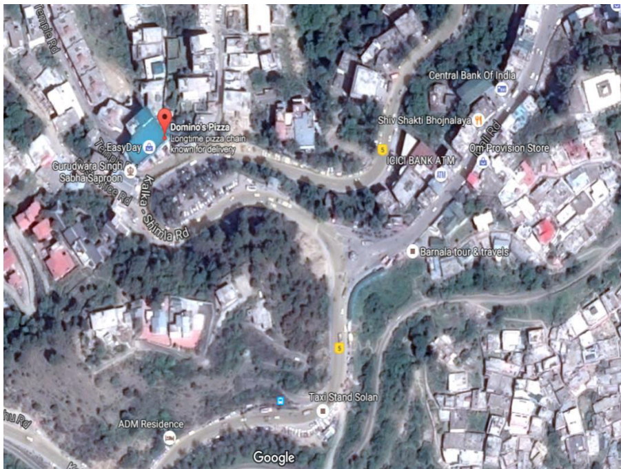
Fig 1.5(e) Aerial view of Solan bypass
