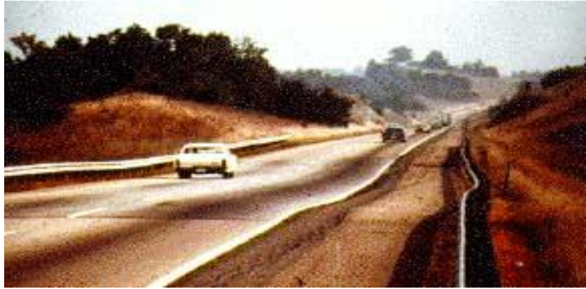
Fig 1.4: Pavement damage due to settling of sub-grade soil.
