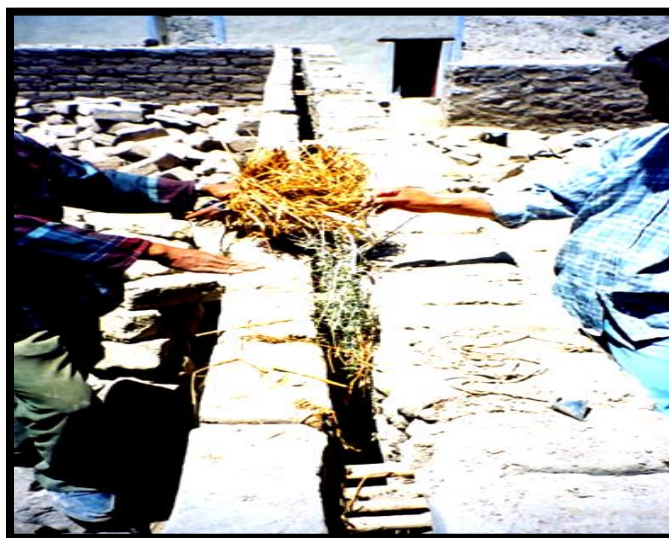
Fig. 5 Traditional construction in Spiti using straw, grass for insulation
