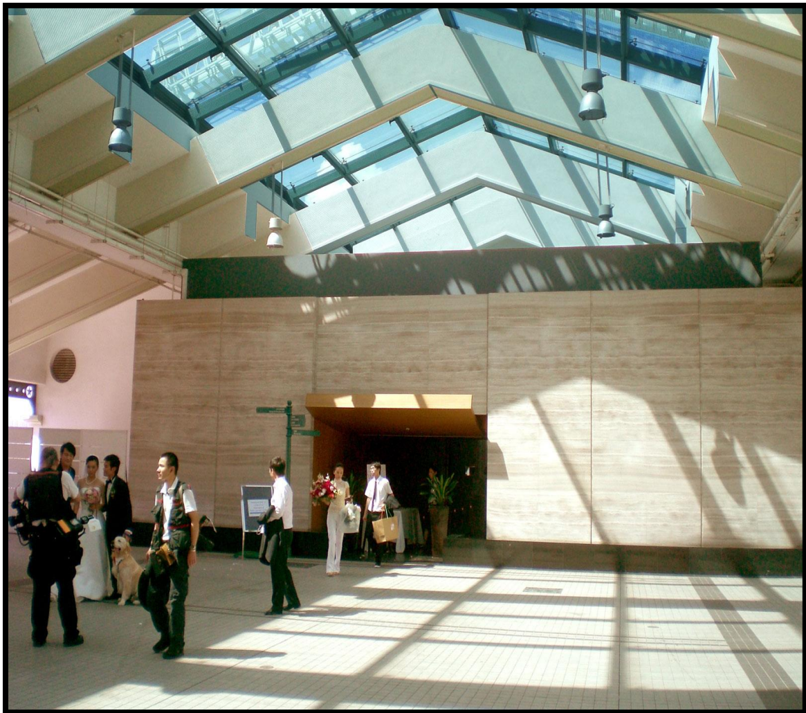
Fig. 3 Skylight in an office
