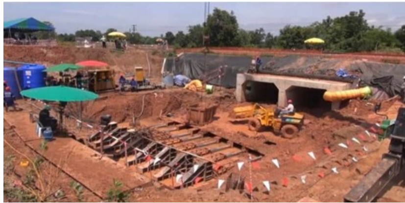
Figure 1.4 Jacking pit and jacked box section (Gordon, E. K., 2015)
