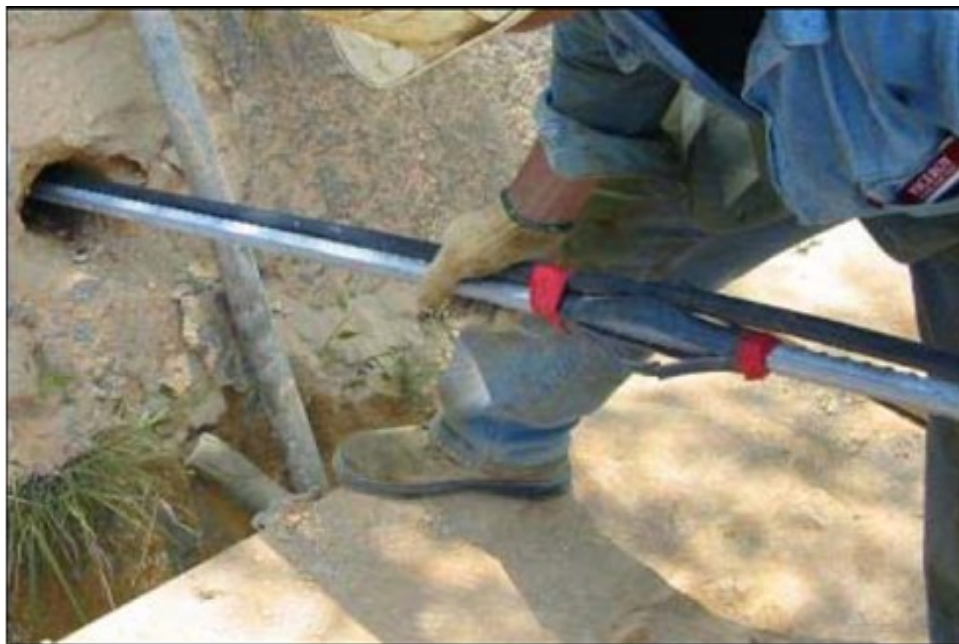
Figure 1.8 Nail installation (Prashant, A., 2010)
