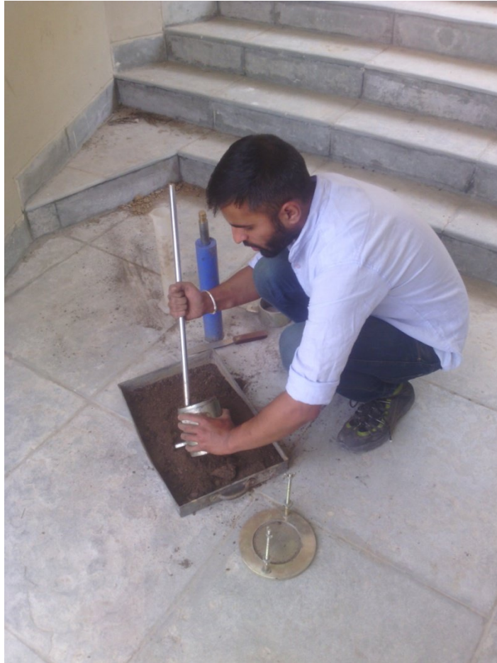
Figure 16 Performing soil compaction
