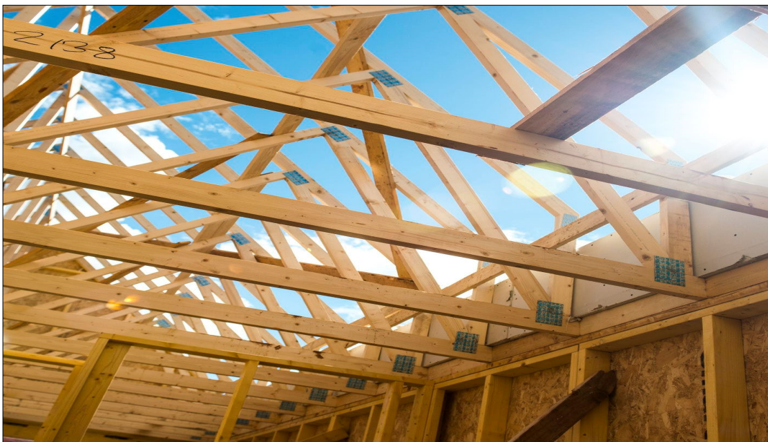
Figure 11: Roof Truss
