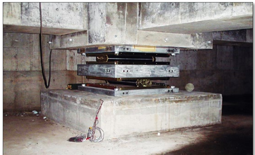
Figure 19 Simple Roller Bearing
