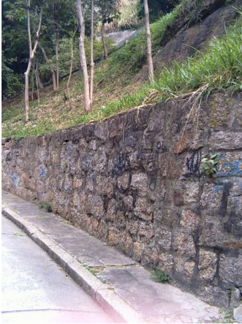
Fig (23) - Retaining Wall
