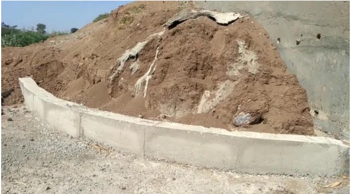
Fig (24) – Toe wall
