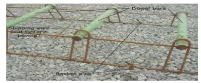
Fig. 3.9: Dowel bar arrangement
