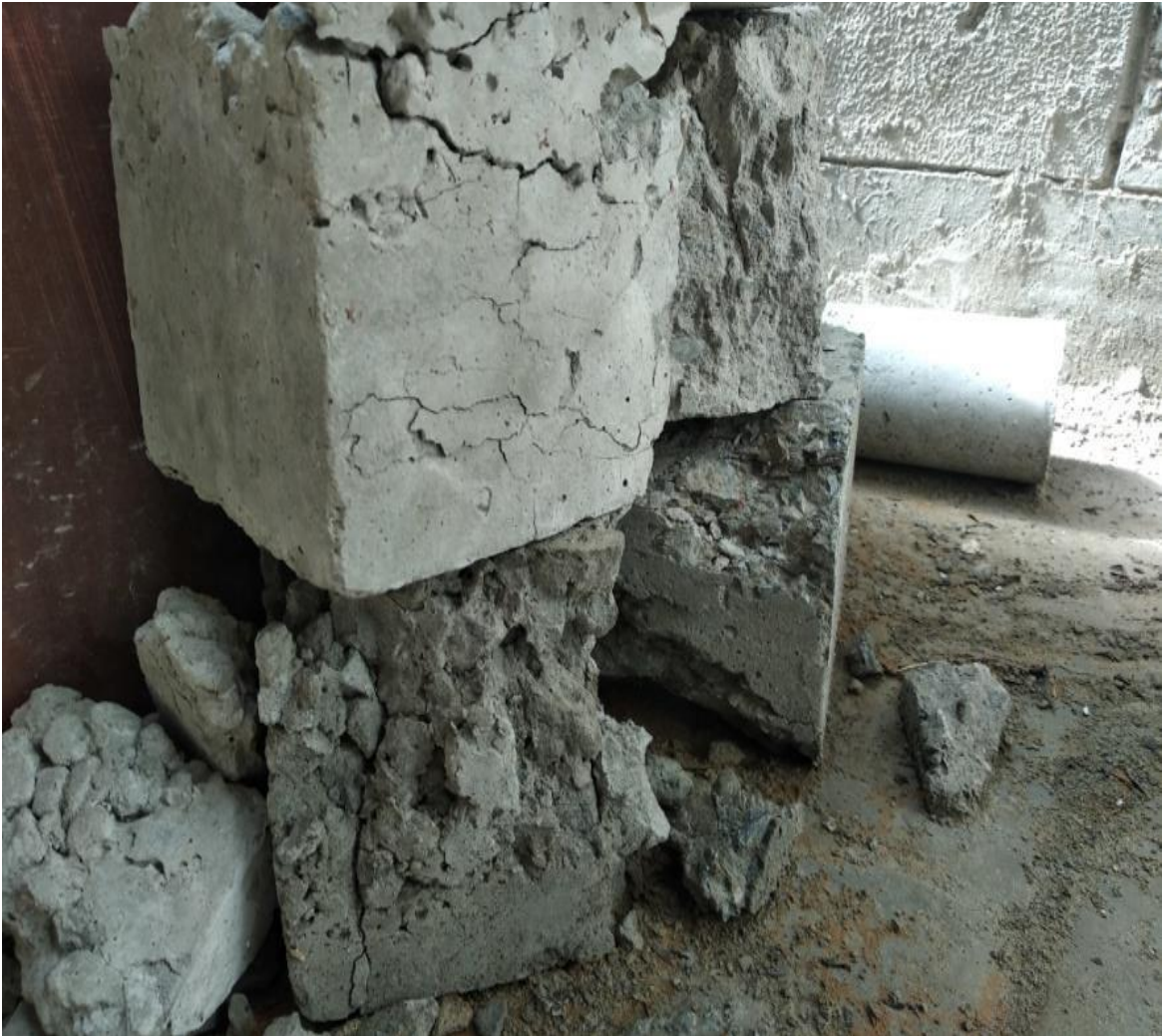
Fig. 3.18 Bagasse cube after cracks under CTM
