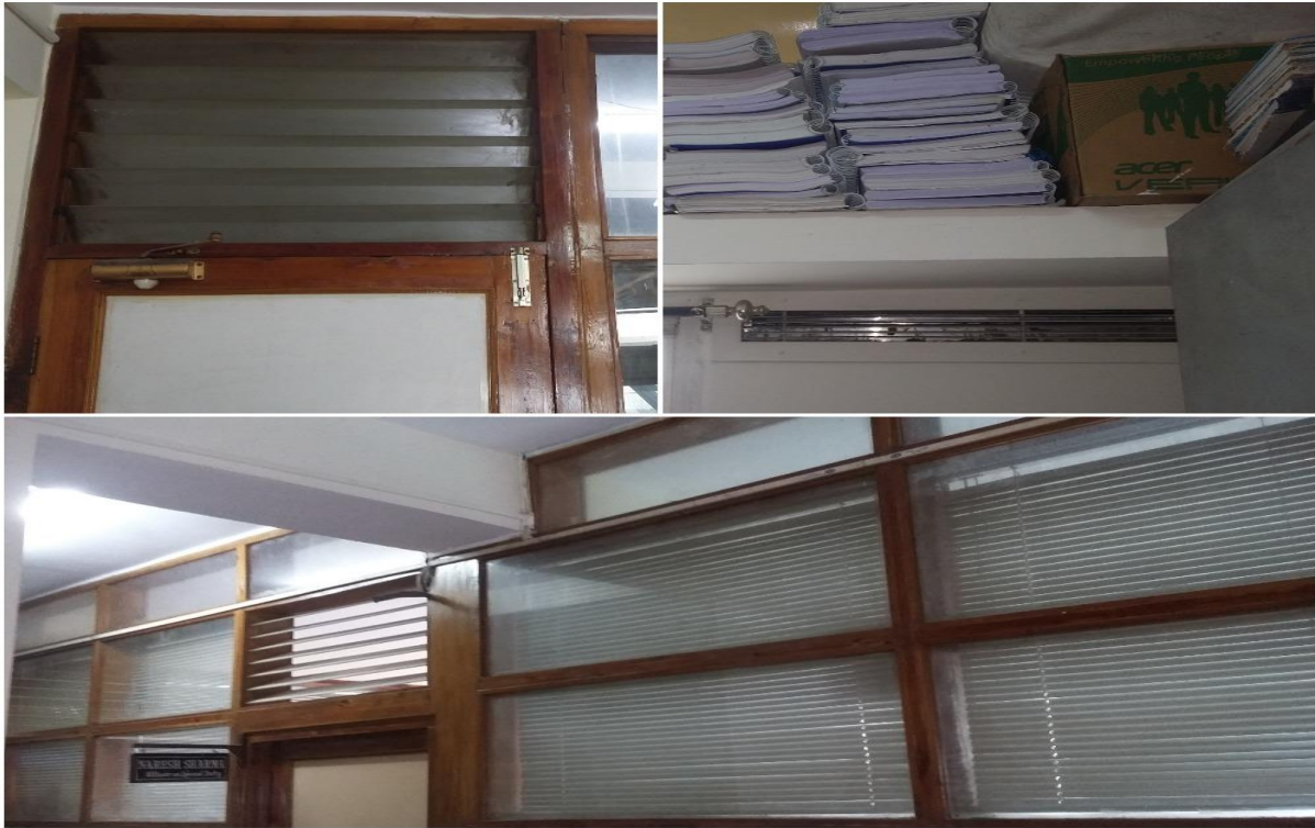
Figure 3: Vents provided for cross ventilation across rooms.
