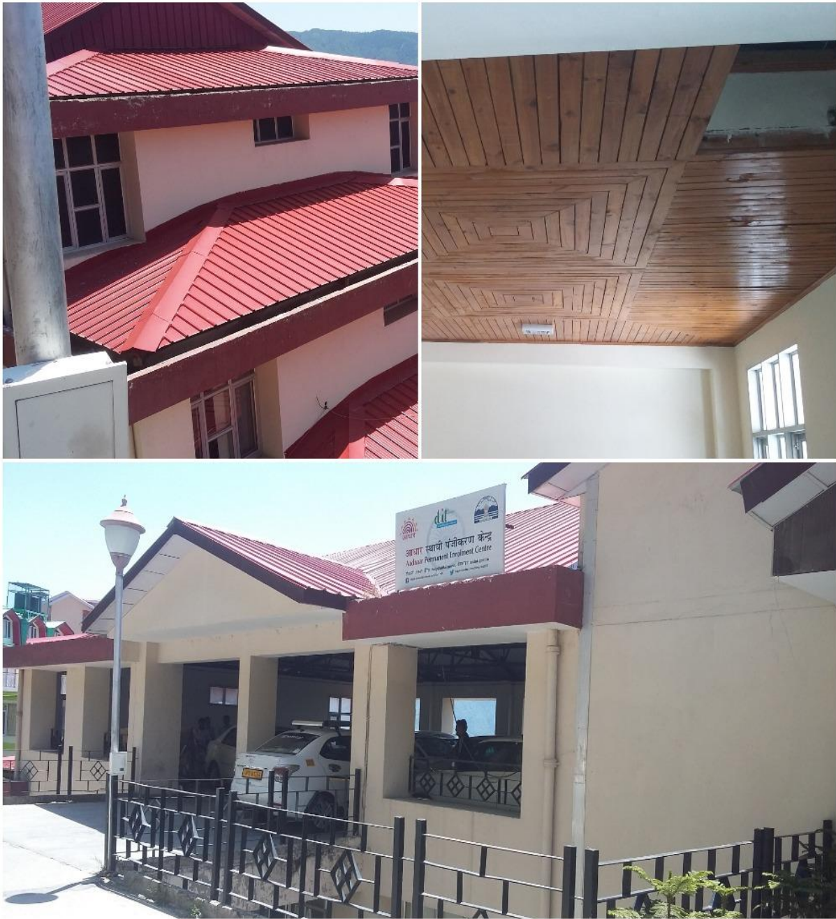
Figure 5: IT Bhawan, Mehli (conventional type of build)
