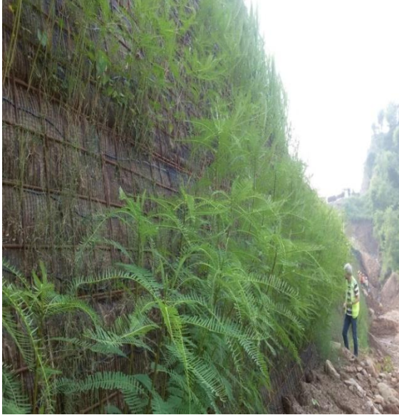
Figure 3.4 (c) Retaining wall
