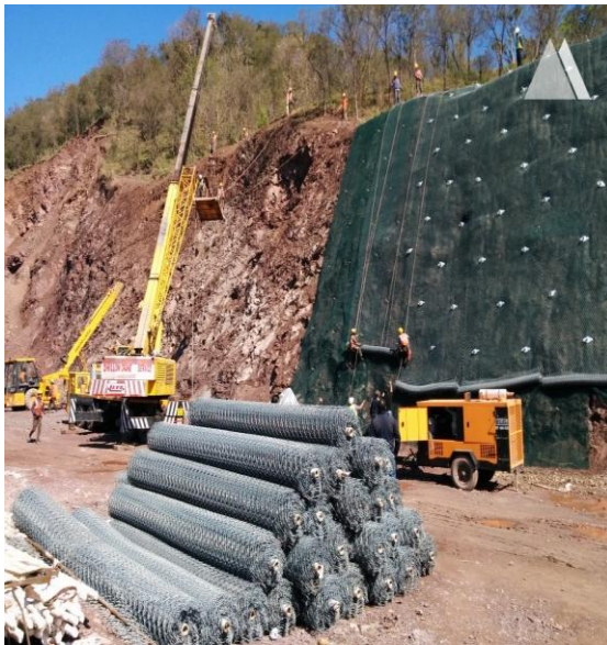
Figure 3.4 (a) Soil stabilization
