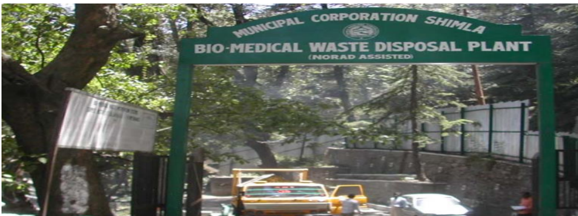
Figure 3.8 Centralized Incineration Facility for Biomedical waste.
