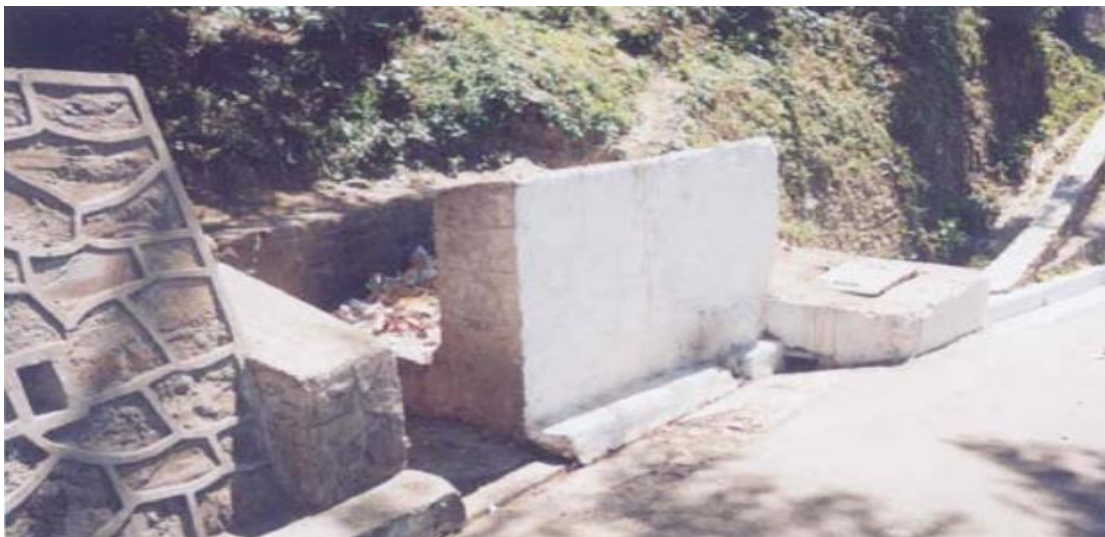
Figure 3.6 A concrete box constructed near mall road Shimla.
