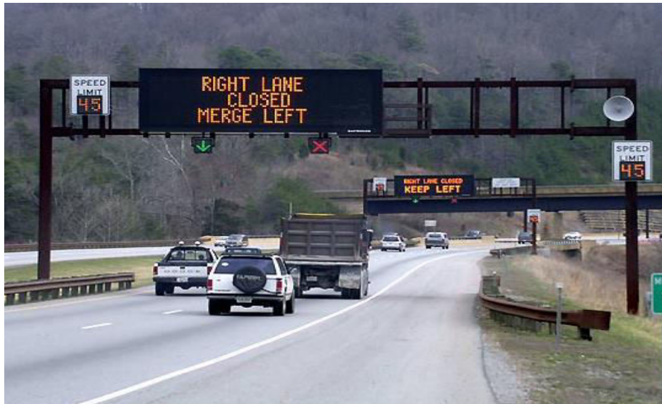
Fig 5.1: Example of ATMS
