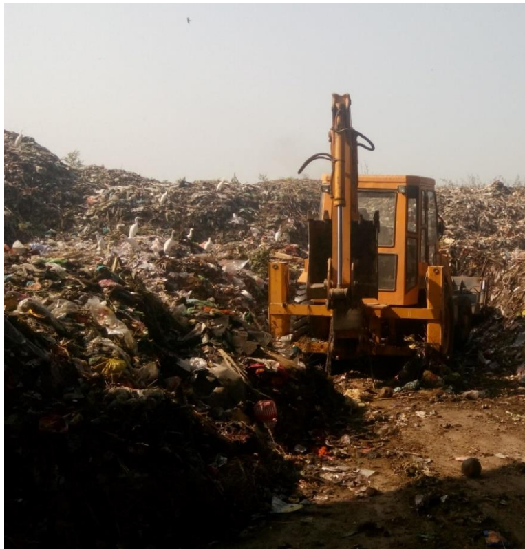
Fig.4.6: Disposal on the Site
