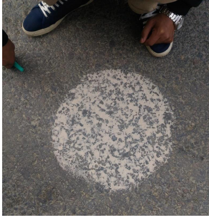
Fig. 4. 16 Sand Patch Test in Domehar road (RR-1)
