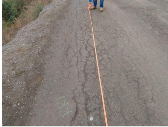
Fig. 4. 8 Mapped cracking
