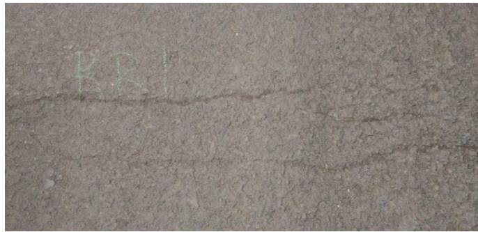
Fig. 4. 9 Transverse cracking
