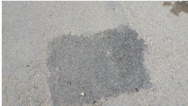
Fig. 4. 7 Patching in Salana Road (RR-6)
