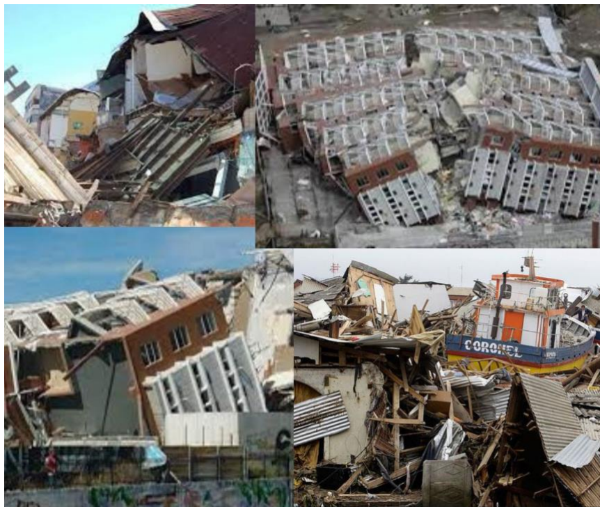
Fig 1.2.4 Disaster in Chile due to earthquake
