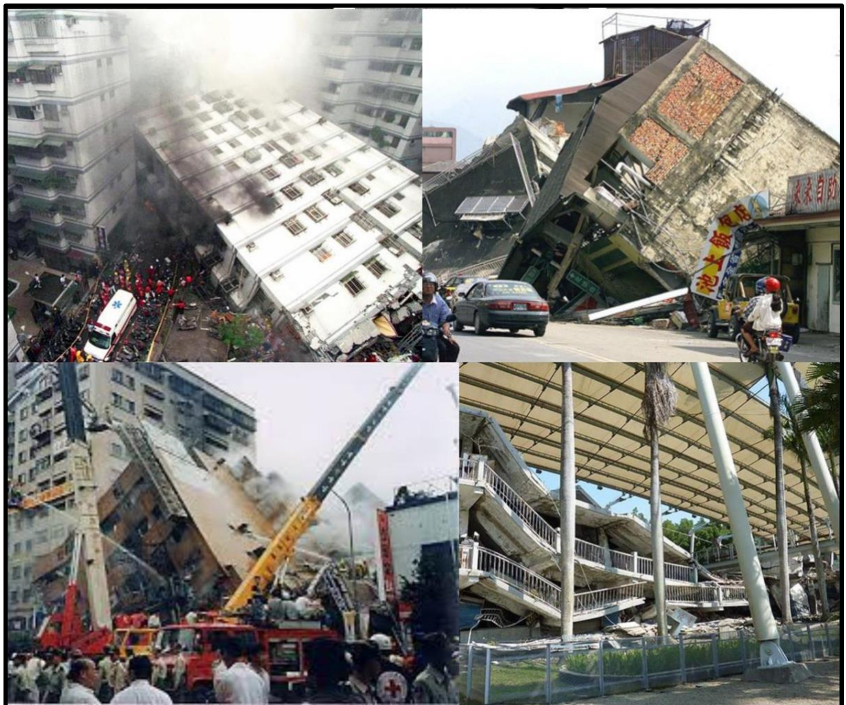
Fig 1.2.3 Damage due to 921 and 1022 earthquakes
