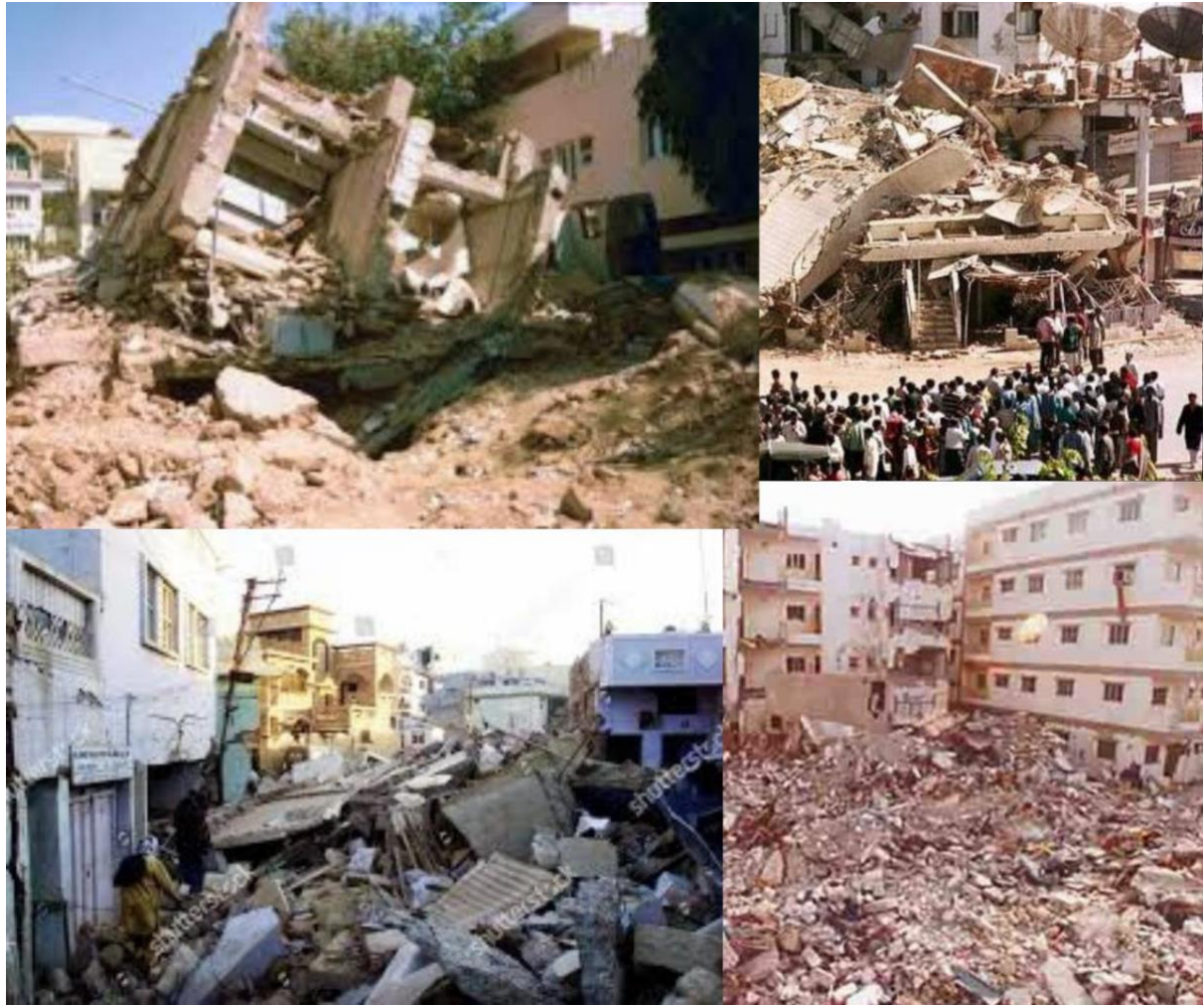
Fig 1.2.2 Damage caused due to Bhuj earthquake
