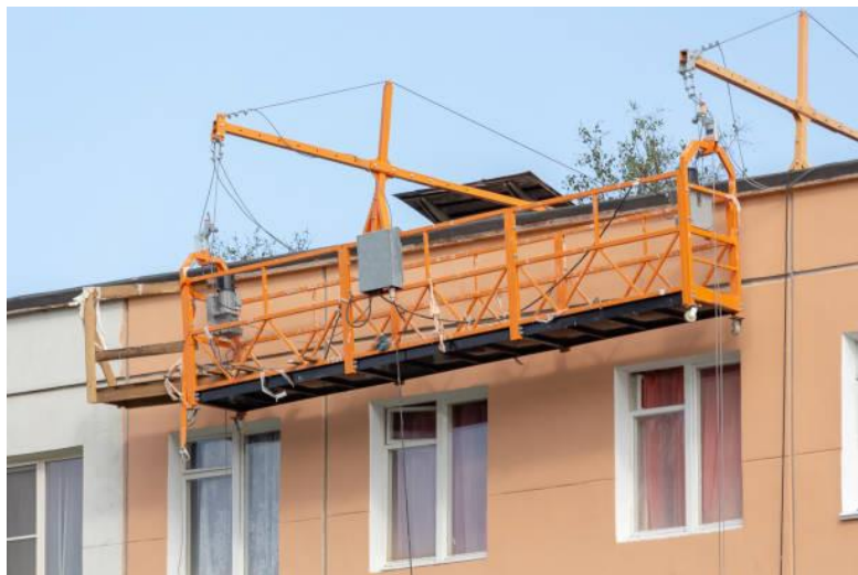
Fig. 3.9 Suspended Scaffoldings
