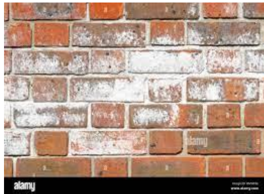
Fig 8. Efflorescence
