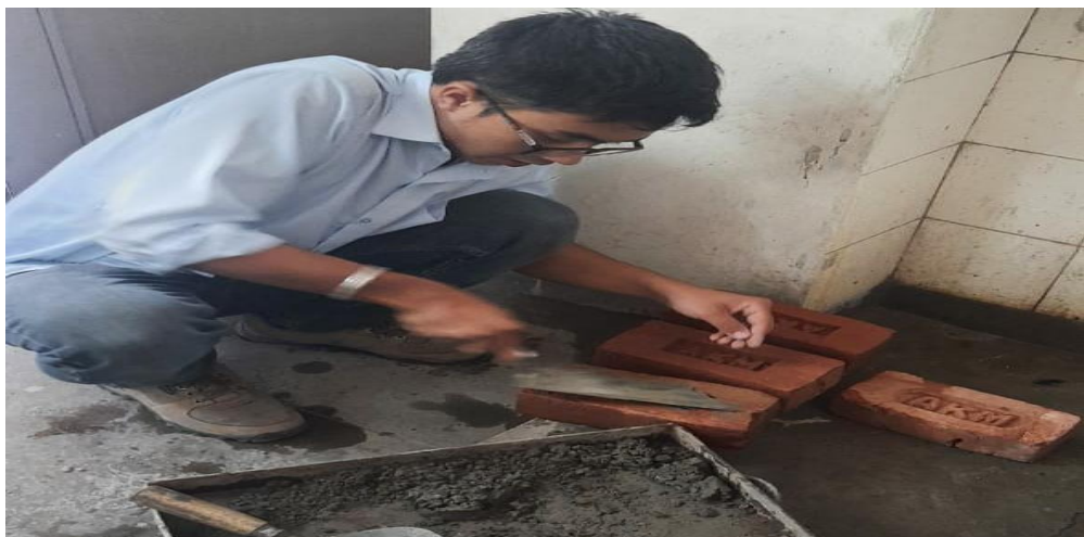
Fig 31. Making surface smooth of red bricks
