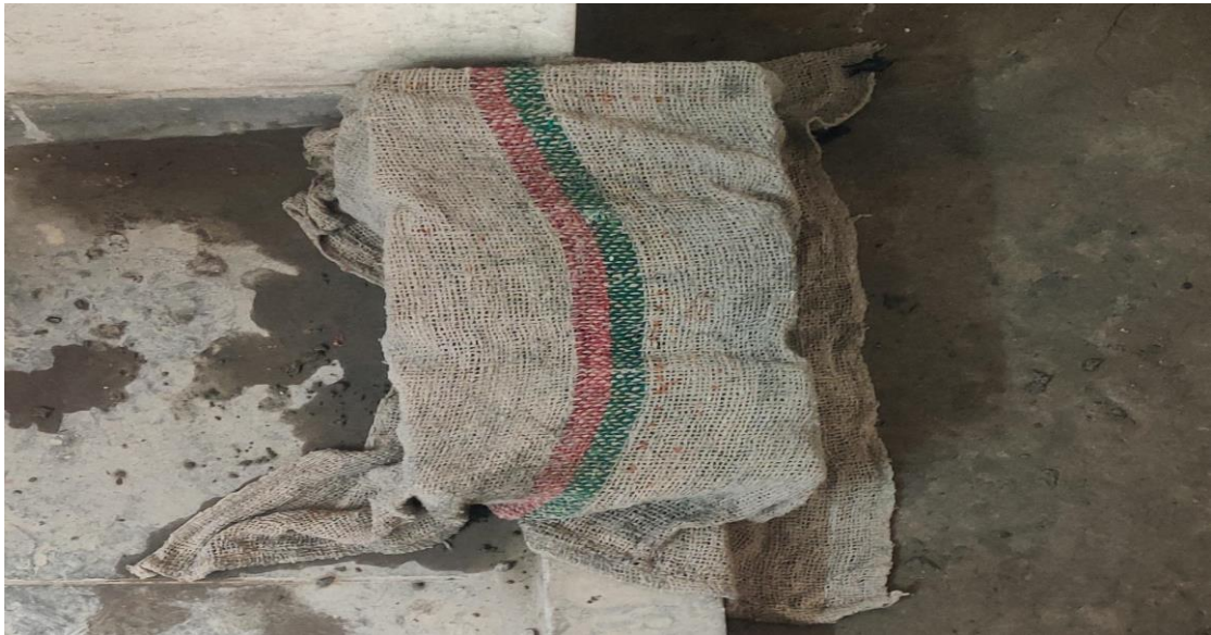
Fig 32. Keeping red bricks in moisture for 24 hours
