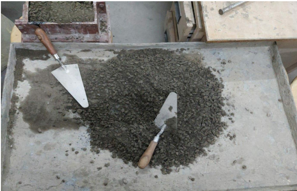
Fig 16. Manually mixed cement and other aggregates
