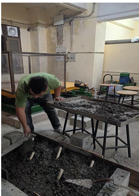
Fig.3.8 (a) Placing concrete in the formwork
