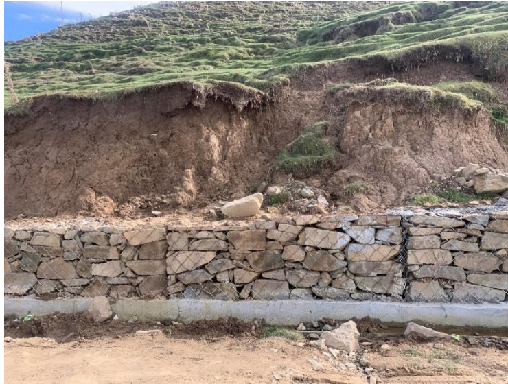
Fig.1.4 Gabion Retaining Wall
