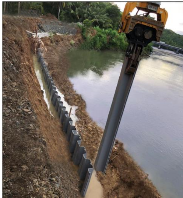
Fig.1.7 Sheet Pile Retaining Wall
