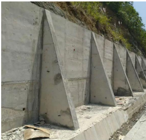
Fig.1.3 (a) Counterfort Retaining Wall
