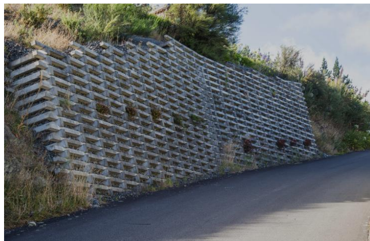
Fig.1.6 Crib Retaining Wall
