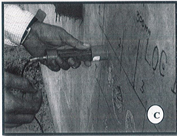
Figure 9: (A) Test surface being made wet; (B) Digital Millivolt Meter; (C) Copper/Copper Sulfate Half-Cell
