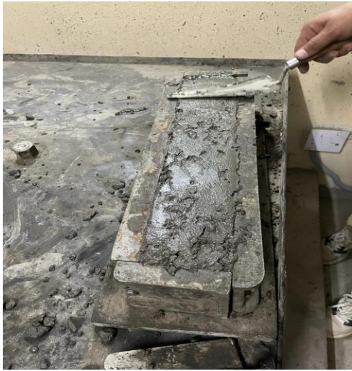
Fig 4.2 Beam during casting
