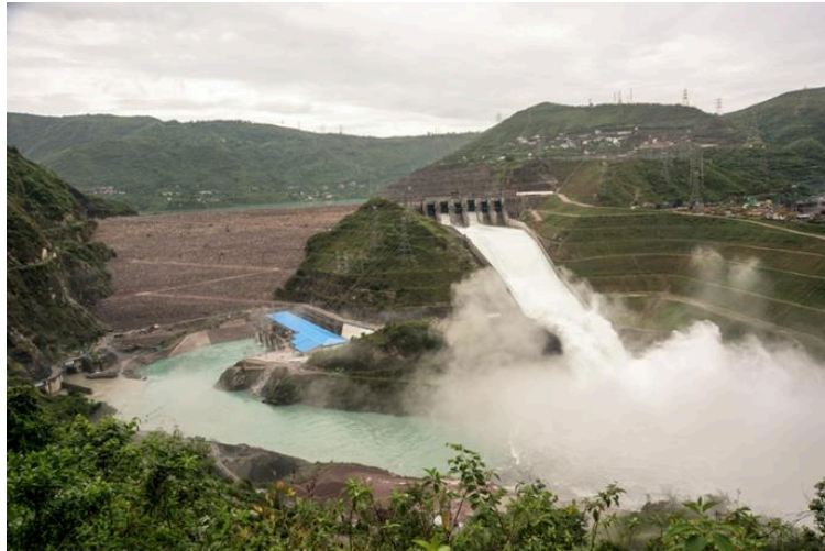
Fig 3.3: Koldam spillway in operation
