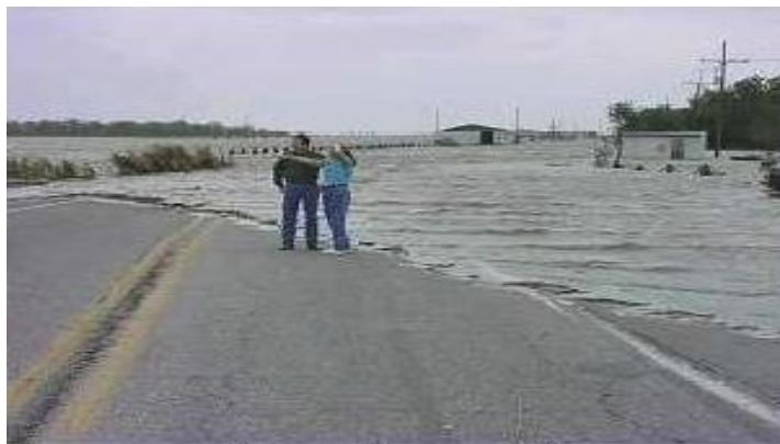
Fig 1.13: Coastal flooding during Hurricane Lili in 2002 on Louisiana Highway
