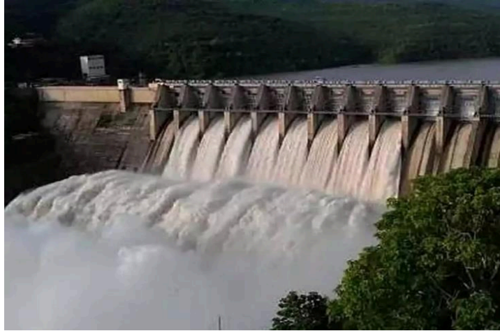
Fig 1.5: Nathpa Jhakri Dam
