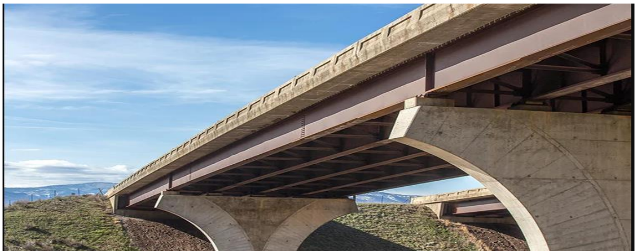
Fig.1.2 Highway Bridge (source Wikipedia)
