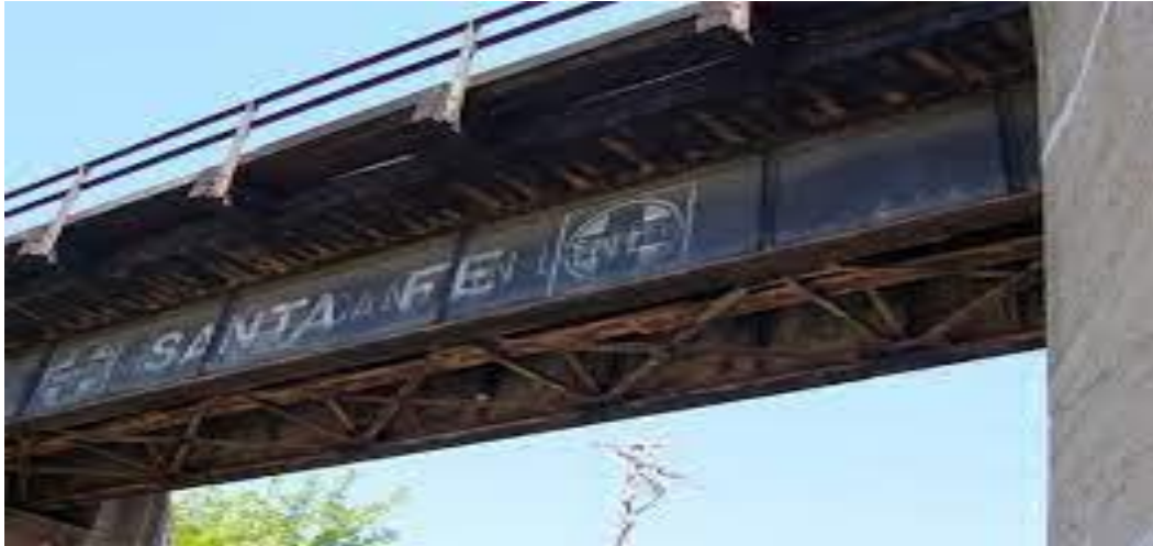
Fig.1.3 Steel Bridge (Source Wikipedia)
