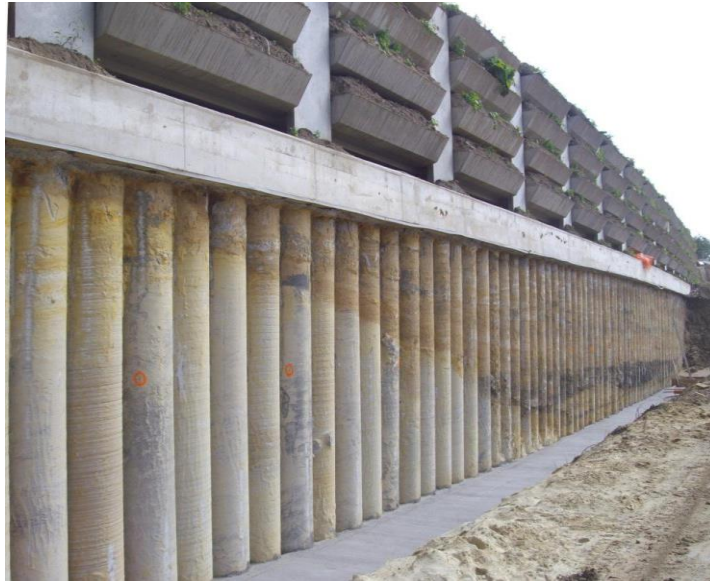
Fig. 1.7 Pilled retaining wall
