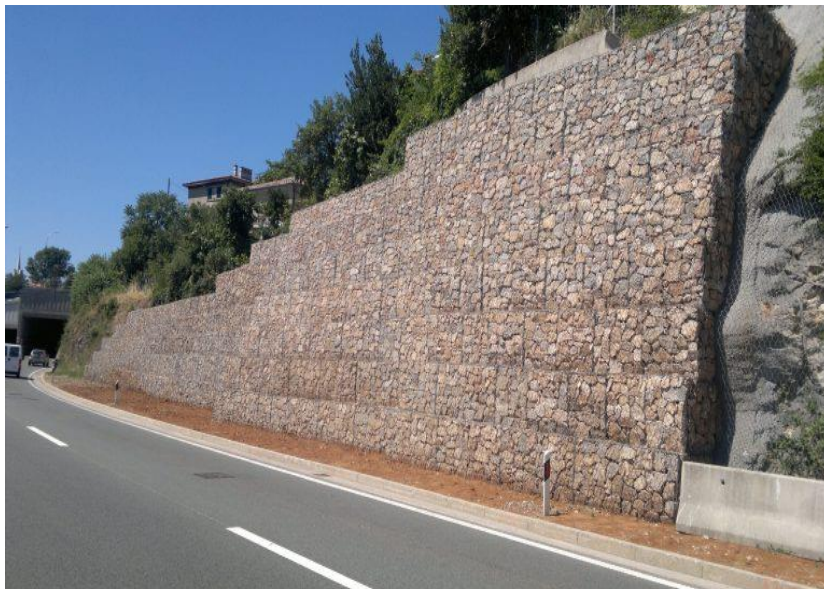
Fig1.8 Gabion retaining wall
