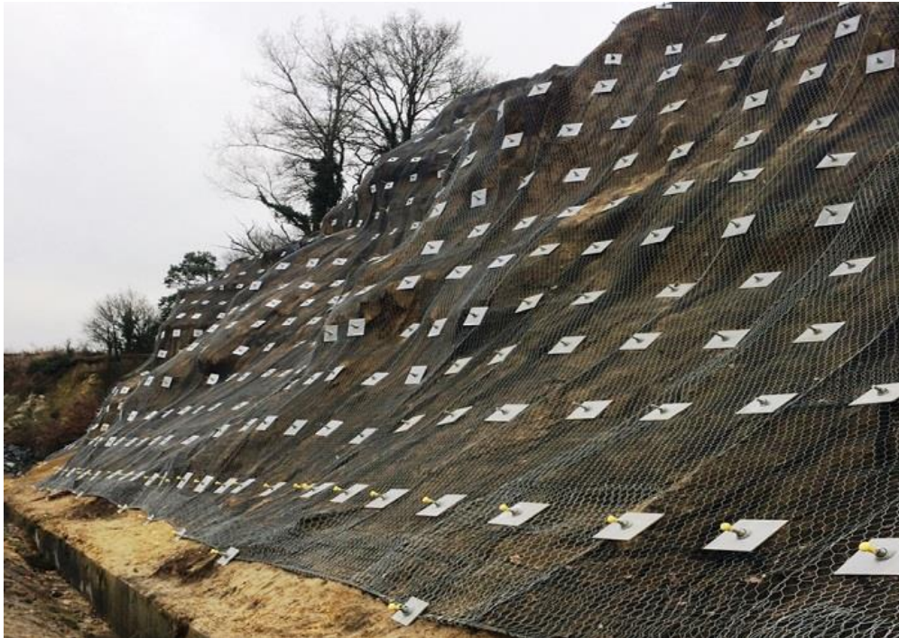
Fig.1.9 Soil nailing retaining wall
