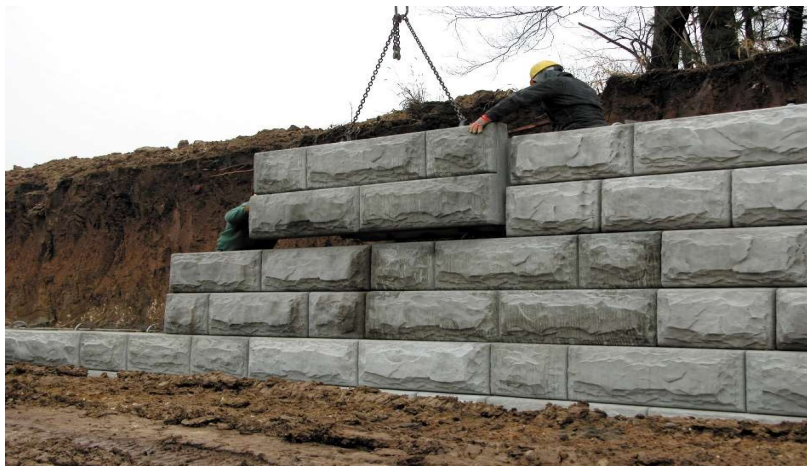
Figure 1.6 Modular Block Retaining Wall
