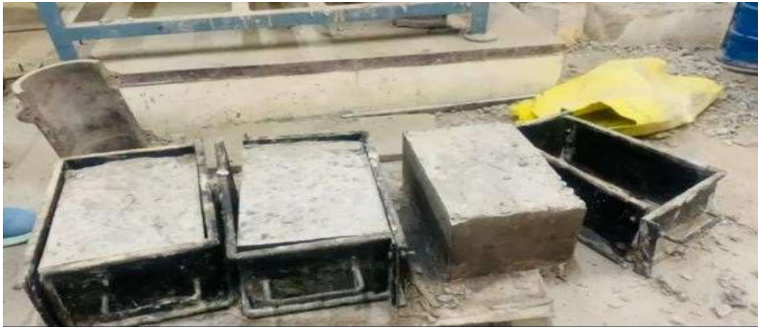
Figure 3.13 Demoulding of blocks
