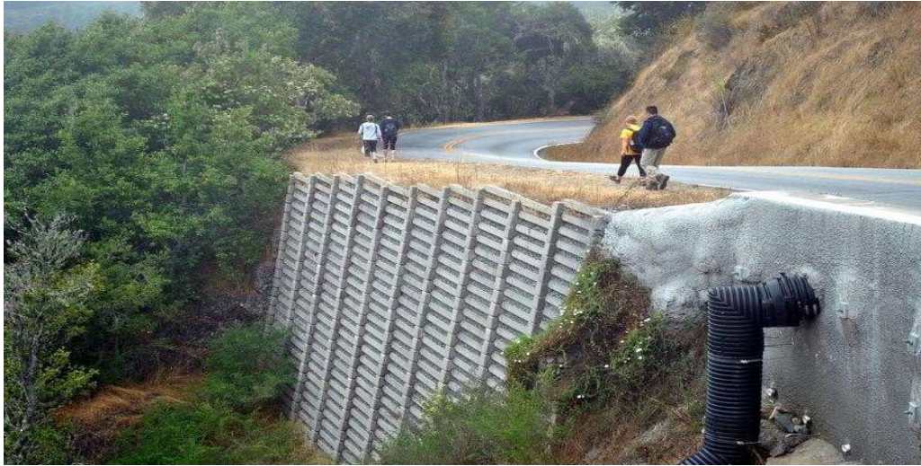
Figure 1.2 Crib Retaining Wall
