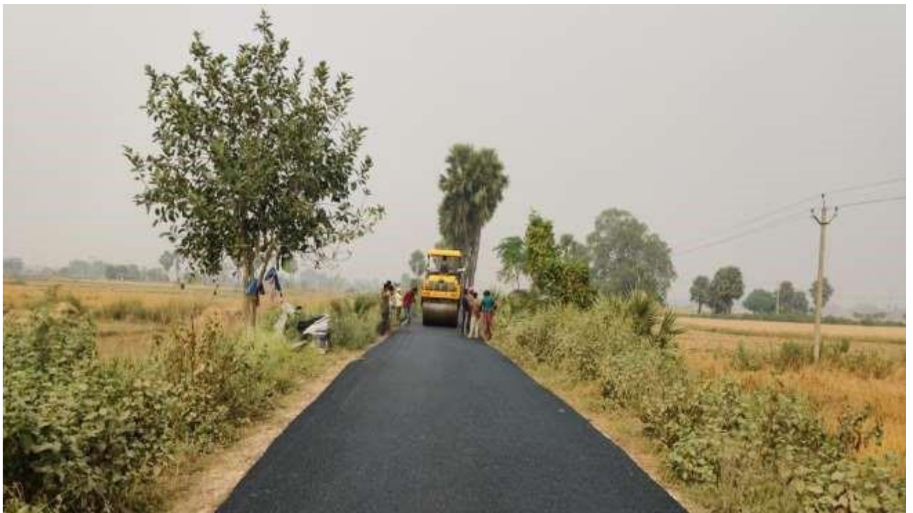
Figure 2.2: Rolling of pavement
