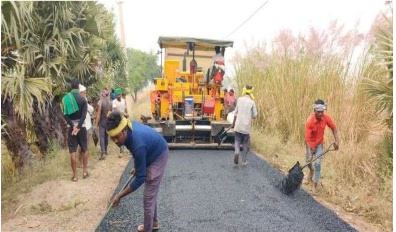
Figure 2.1: Laying of asphalt using paver
